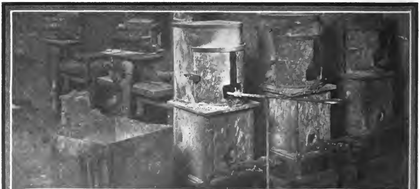
Fig. 22— Salt furnaces, used in heat treating work at the plant where Diamond chains are made
